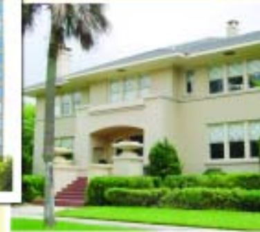
Jacksonville - Copeland Office
